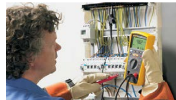
Insulation test at a distribution panel
